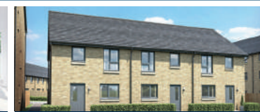
A range of apartments and houses
